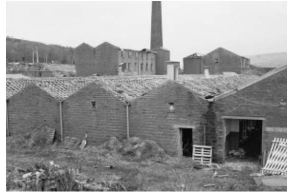
View across weaving shed from the west showing the two three storey buildings beyond and the corner of the modern extension on the right.
