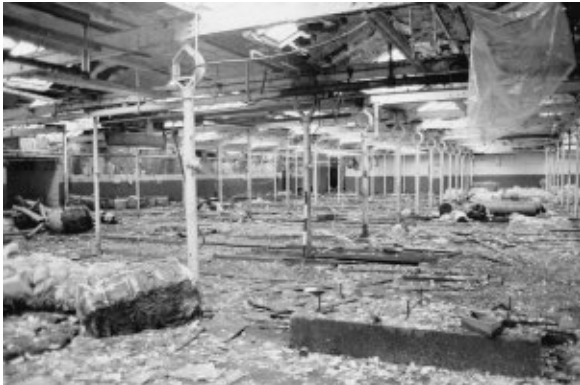
View from the western end of the weaving shed looking along the central line of columns which held the drive shaft.
