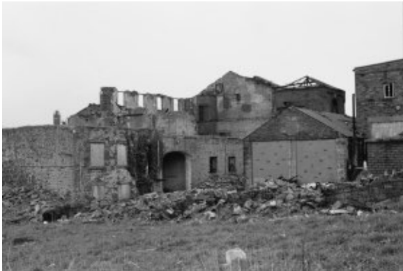
Looking south west at the north face of the rear three storey building and the boiler house.
