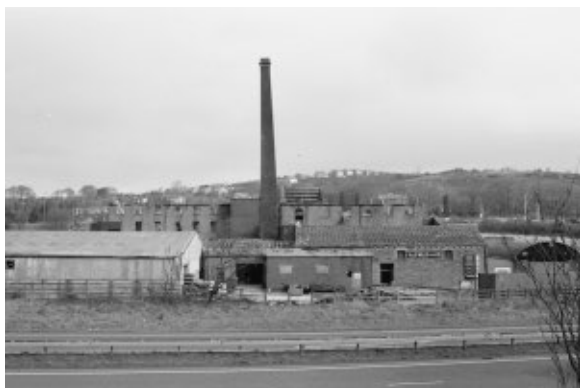
View of the mill site from the south.
