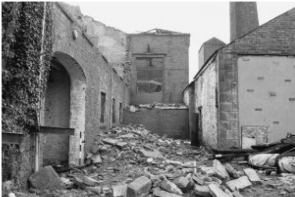
View along north face of rear three storey building with brick extension for horizontal steam engine and boiler house on the right.
