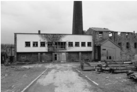
Looking south at the office building.
