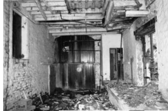
Looking south through the archway under the rear three storey building.
