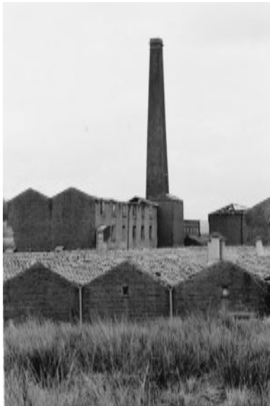
View across weaving shed from the west showing brick lift shaft on front three storey building and extension to engine house on rear three storey building.
