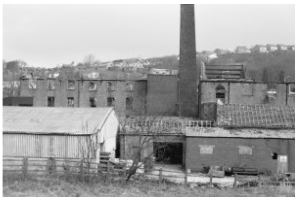
View from the south showing the engine house window centre right and the lift shaft next to the chimney.
