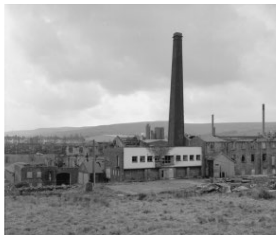
General view from the north east.
