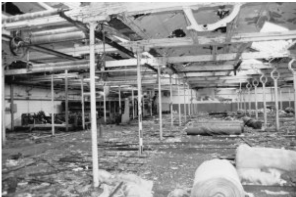
View looking to the west in the weaving shed showing some of the counter shaft hangers and carriers.
