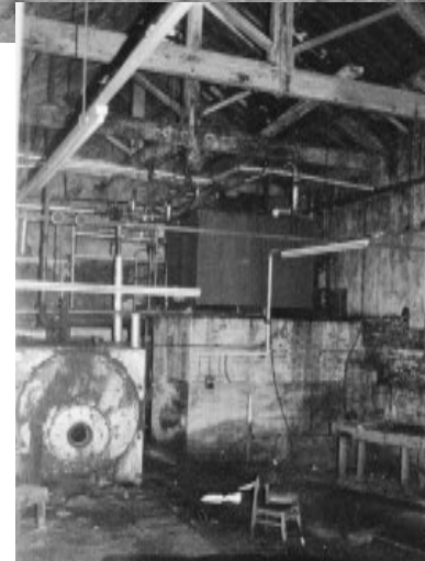
Looking west inside the boiler house.
