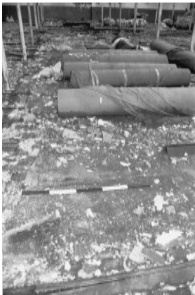
View looking to the west in the weaving shed showing cast iron machinery fixing slots in the floor.
