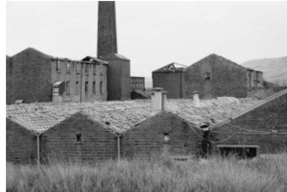
View across weaving shed from the west showing the two three storey buildings beyond and the corner of the modern extension on the right.
