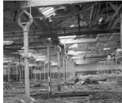
Looking east from the west wall of the weaving shed.
