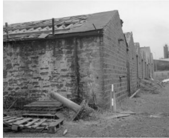
North west corner of the weaving shed showing the water-shot stonework of the west wall.
