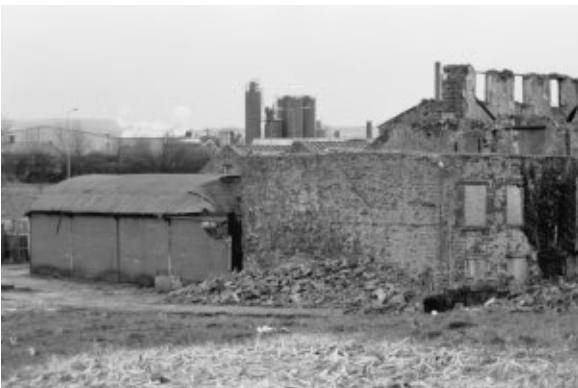
Looking south west at the east face of the rear three storey building and the metal-framed building.
