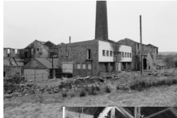
Looking southwest at the office block.
