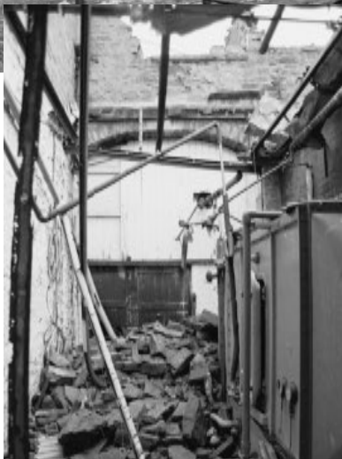
Looking north at the archway through the rear three storey building.
