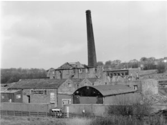
General view from the south east.
