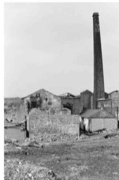
View of the rear three storey building from the east with the boiler house and new office block on the right.
