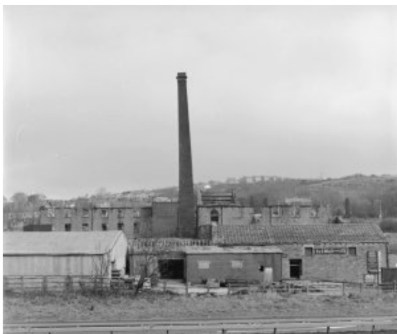
General view from the south.
