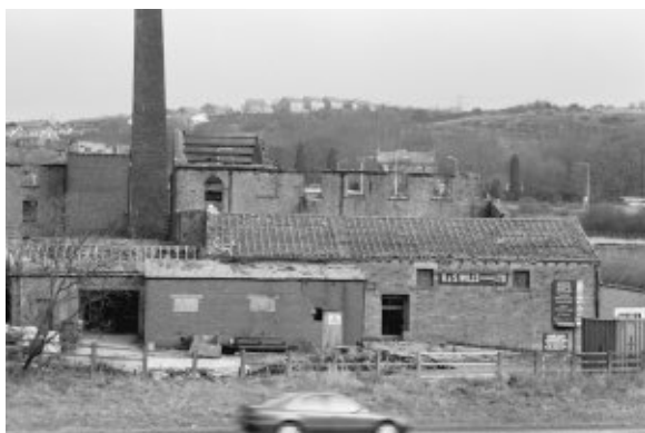
View of the 1907 extension and the rear three storey building from the south.
