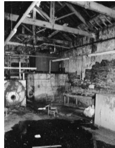
Looking west inside the boiler house.
