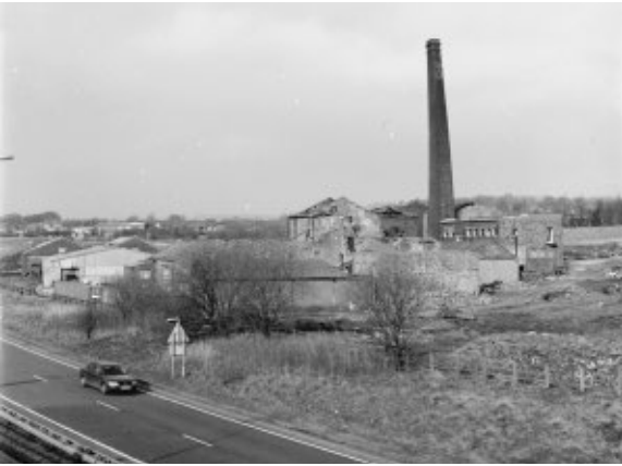
General view from the south east.
