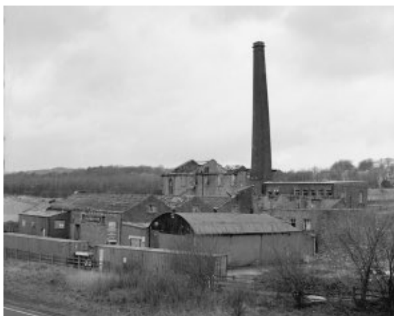
General view from the south east.
