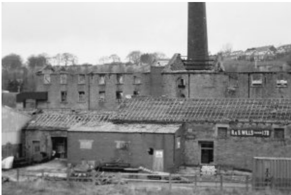
View from south showing engine house window on left side of rear three-storey building and location of date from former cottage and 1907 commemorative stone.
