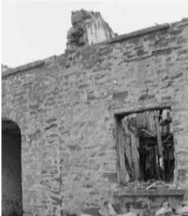
North face of the rear three storey building showing the joint between the two phases of construction. The archway was part of the second phase.
